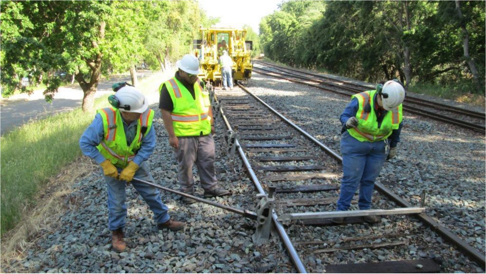
Mike W. cranks on the jack as Heather monitors the level for establishing a proper super-elevation
