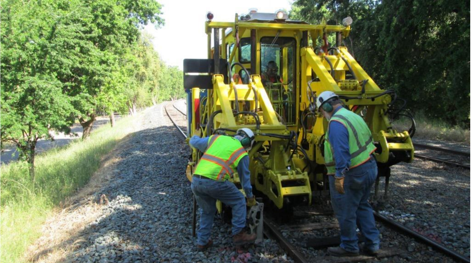
Mike W. removes a jack as the tamper approaches
