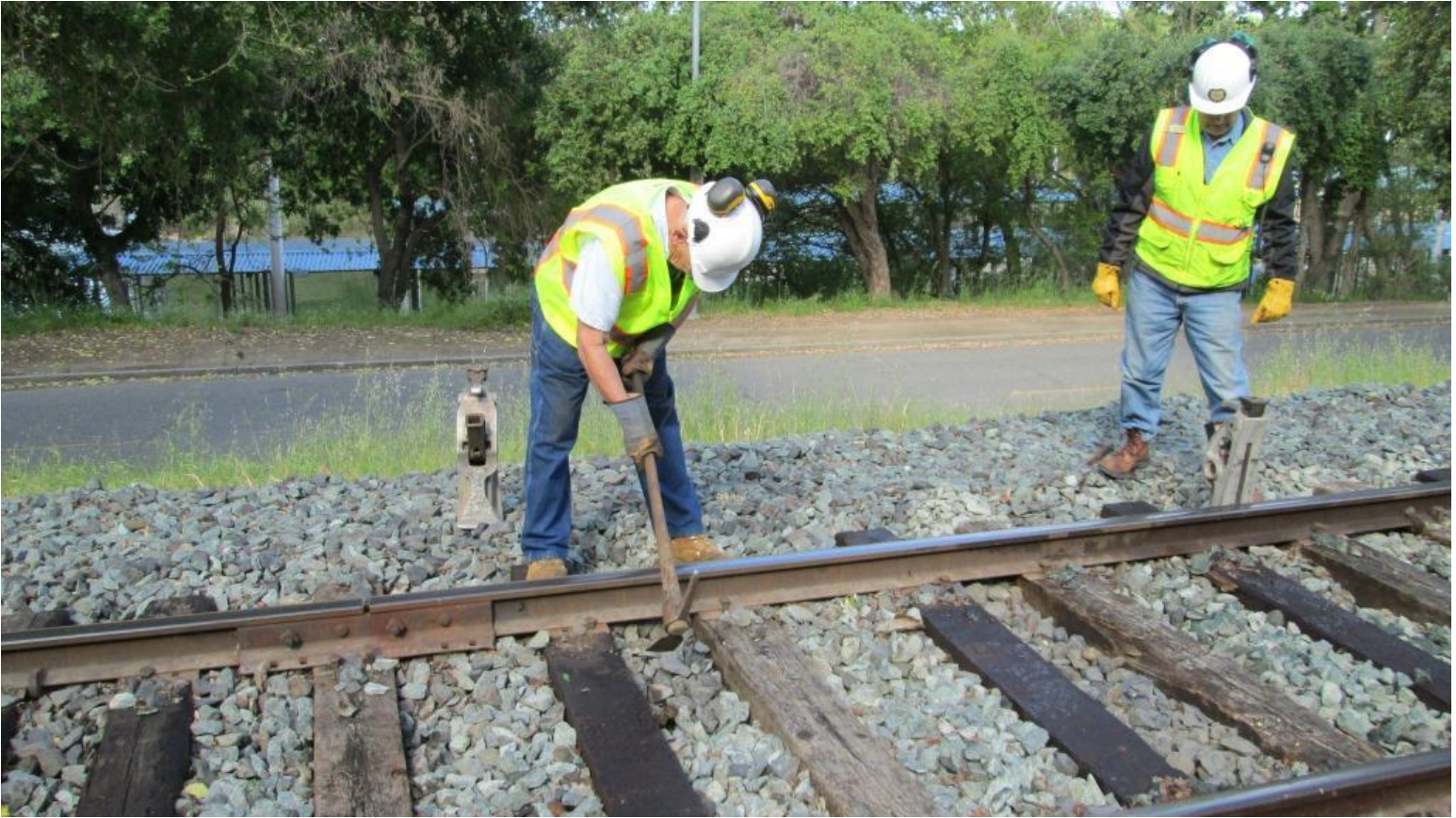
Clem knocks-out enough rock from under the base of the rail for the jack to fit
