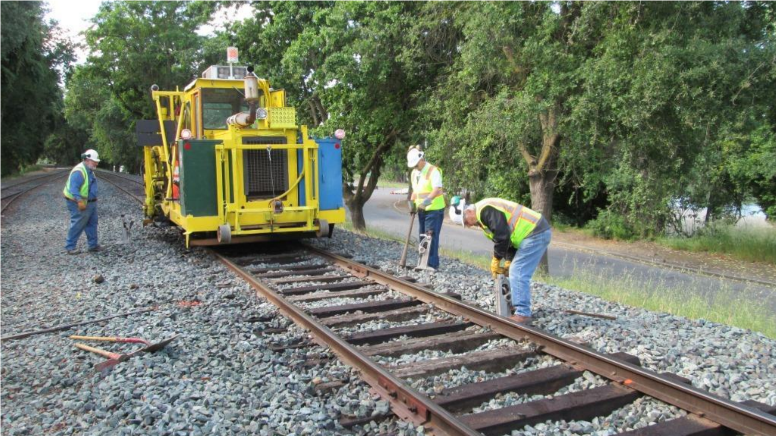
Frank unloads jacks off the tamper while Clem and Mike W. set them in place
