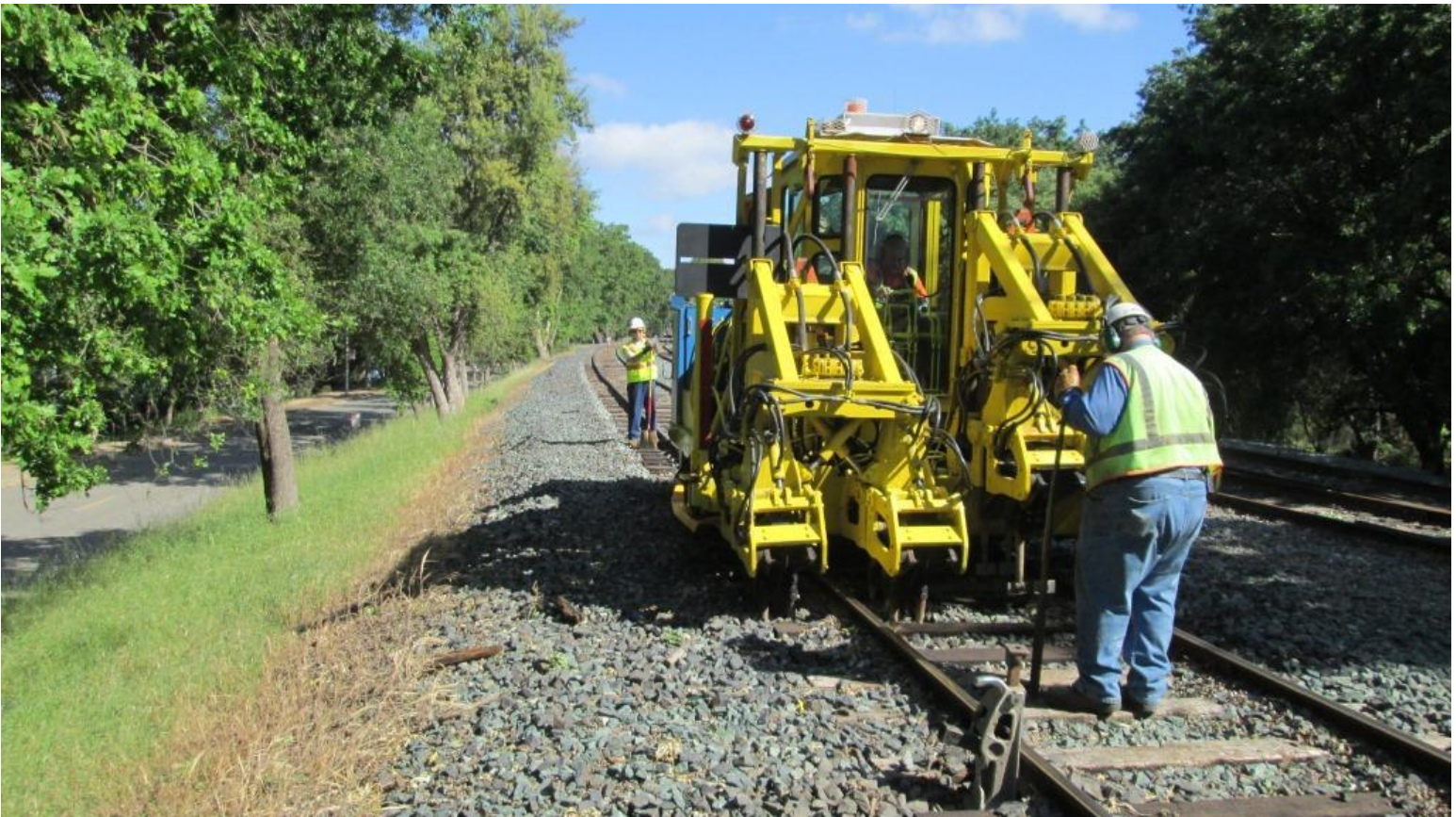
Mike F. operates the tamper while Frank guides from the ground
