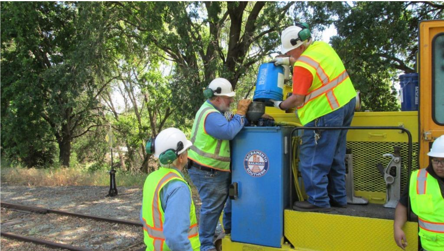
Frank and Harry add hydraulic fluid to the tamper
